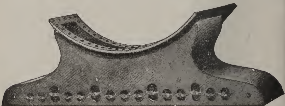
FIG. 15. STEEL SADDLE OF BONSON BOILER.
